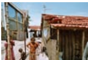
Figure 5: Vaira Maligai temporary shelter, with a vast majority of inhabitants Dalits and Adivasi. The roofing has warped and the mud washed away from the thatch so that the rain pours straight in and floods the shelters. September 2005
